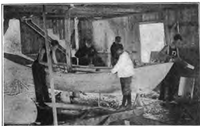
Boat Building at Camp Durrell
